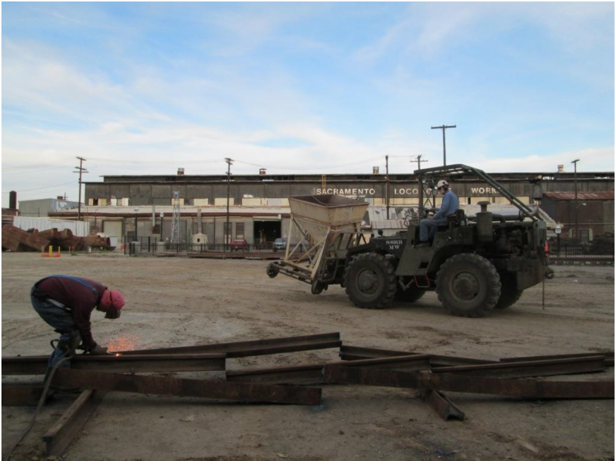
Cliff torch-cuts scrap rail while Alan moves a ballast hopper with Big Green
