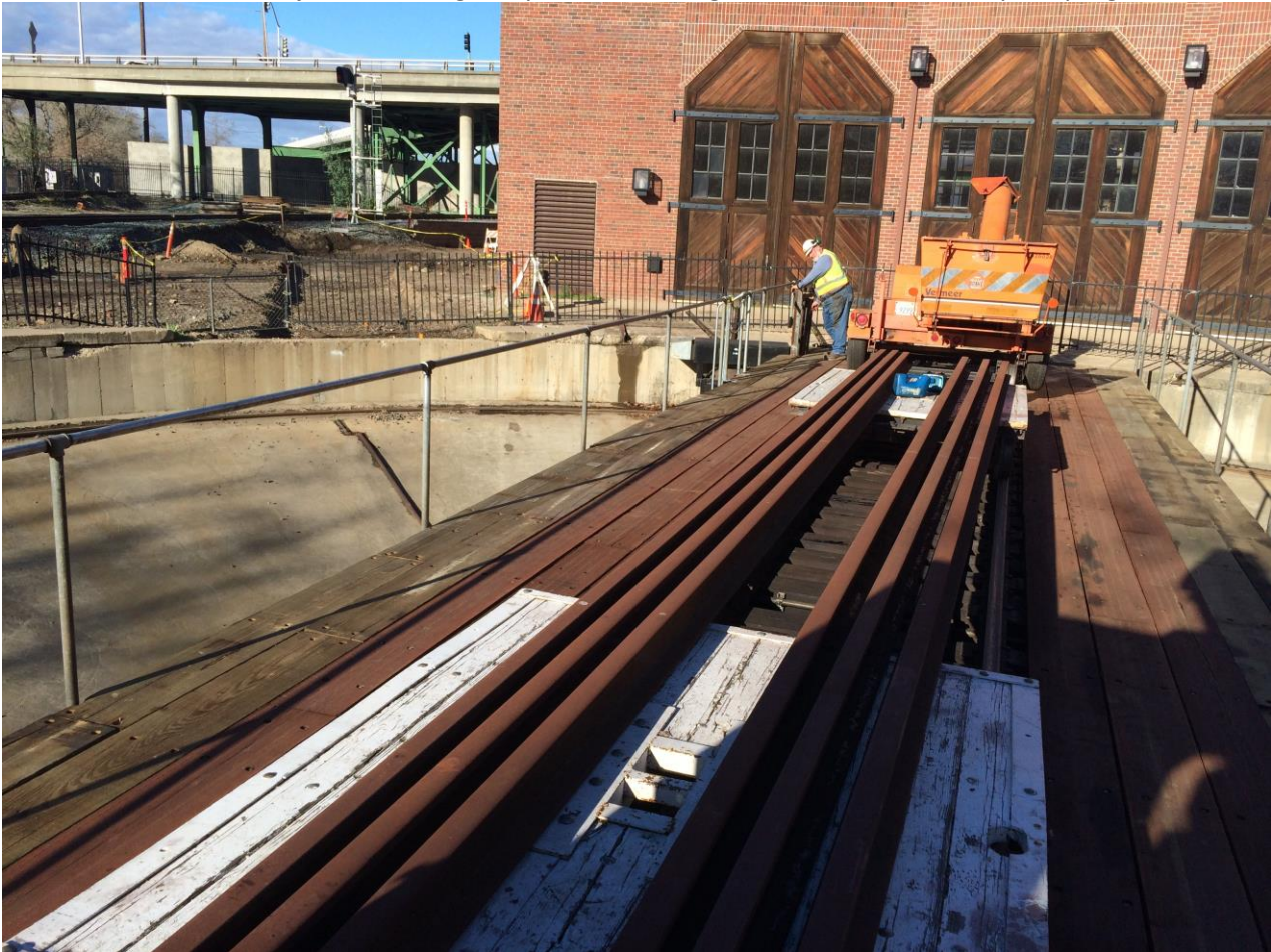
Frank spinning the man-lift consist complete with rails to be used for the new Whisker Track
