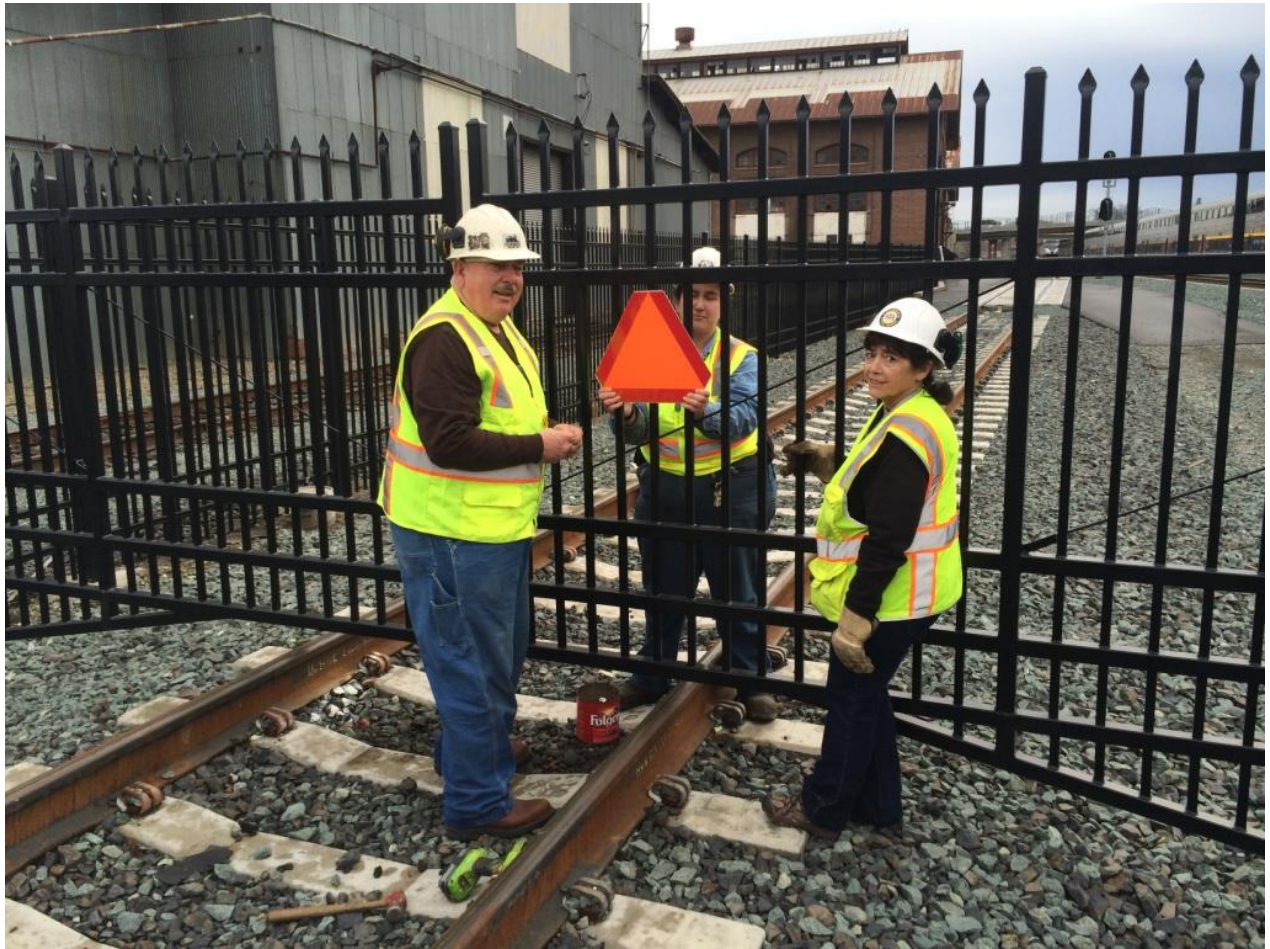
Harry, Heather, and Pam install the highly reflective safety reflectors on the east gates of the 560 Track
