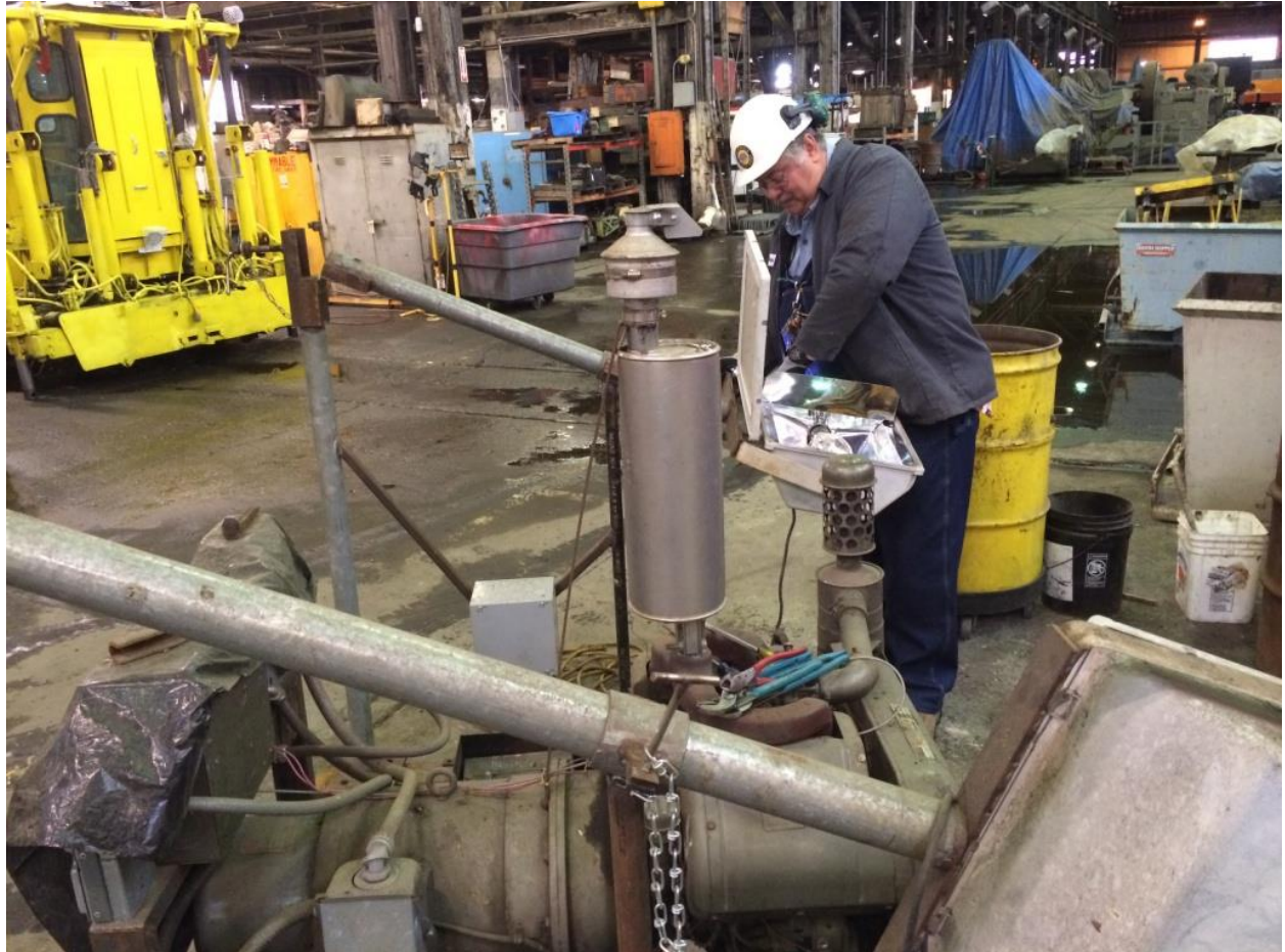
Chris bringing light to darkness by wiring the new MOW night-light...
