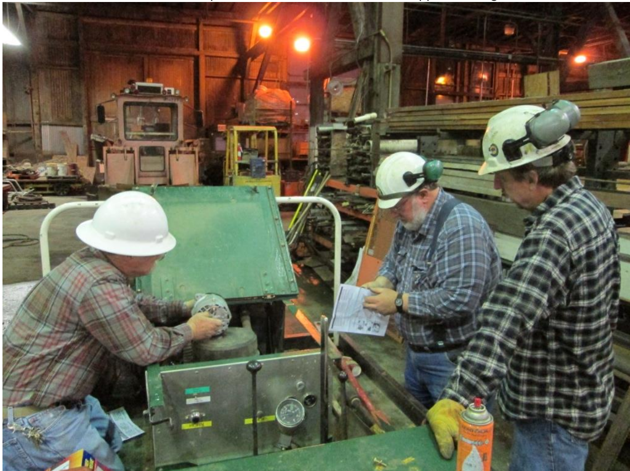
Mike H. and Frank work on the alternator conversion of the A-6 motorcar
