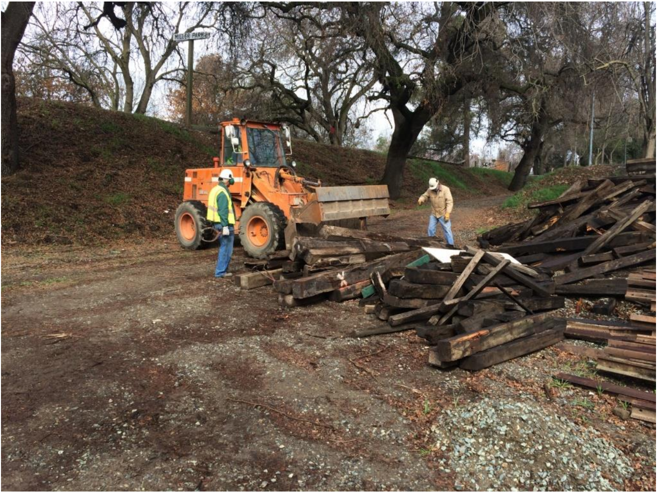
Steve and Alan direct Frank in the loader to grab some extra-heavy dead ties
